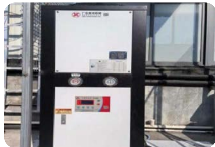
Industrial circulating water chiller
