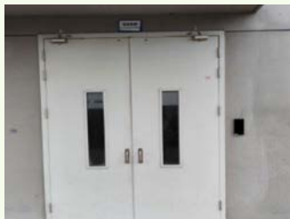
Air compressor housed in a separate room for noise isolation
